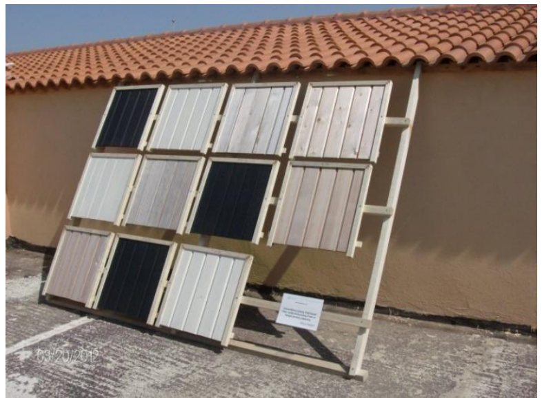
Outdoor cladding-test area at the WST lab
